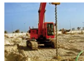
Auger / De-watering drill
